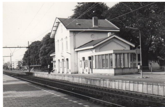
Foto 10 Station Vught in 1965 (bron Jan Siepel)
