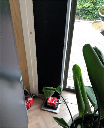
ZT47, begane grond in hoek lobby fitnessschool
